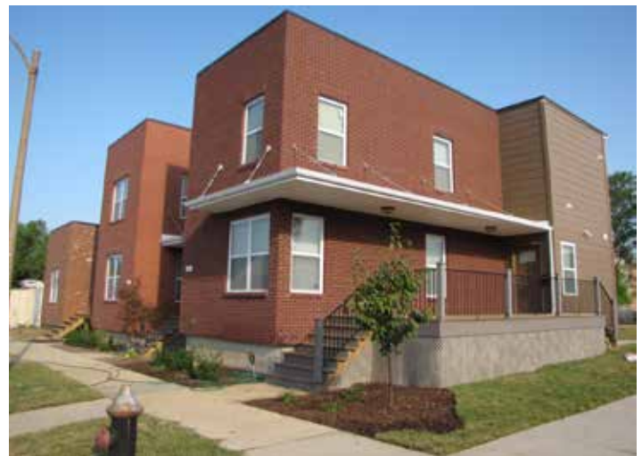
Photo: Courtesy of Habitat for Humanity Saint Louis This property is one of many Habitat for Humanity projects that benefitted from NMTC financing.
